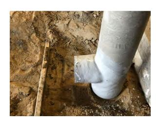
2. Peel the embedded peel-ply tape from the inside of the Grip Seal clamp and slide the clamp assembly over the end of one of the duct sections to be joined.
