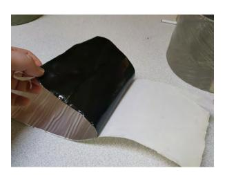
7. Wrap the gasket around the joint area with the silver foil backing placed to the outside. Align the gasket evenly across the joint area with the 2" overlap located at the top of the duct.
