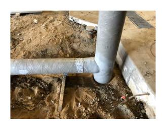
4. Align the cleaned duct sections, making sure that the joint area cannot move during the clamp placement. Small gaps at the joint area are acceptable.
