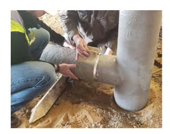
12. Finished Grip Seal clamp installation. Pressure test duct system when completed to check for leaks.
